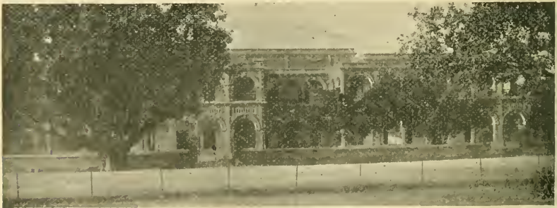
LOIS L. PARKER HIGH SCHOOL, LUCKNOW, INDIA
